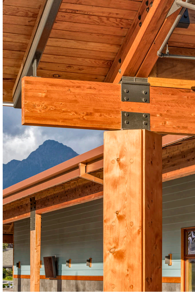
Alaska Yellow Cedar column wraps at Sitka Harrigan Centennial Hall
