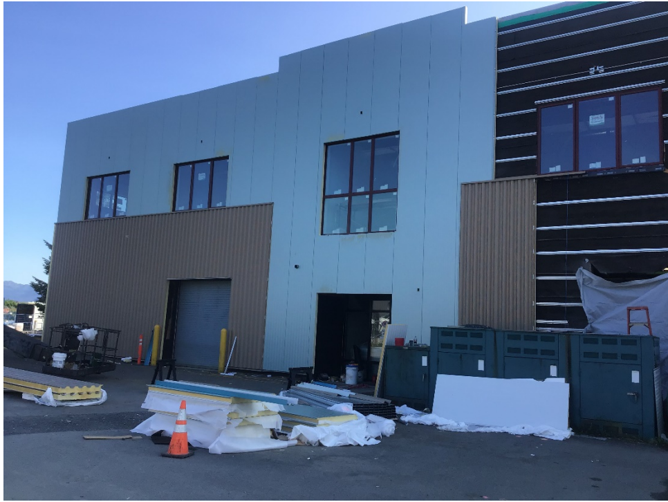
Insulated Wall Panels on Sitka Waste Water Treatment Plant
